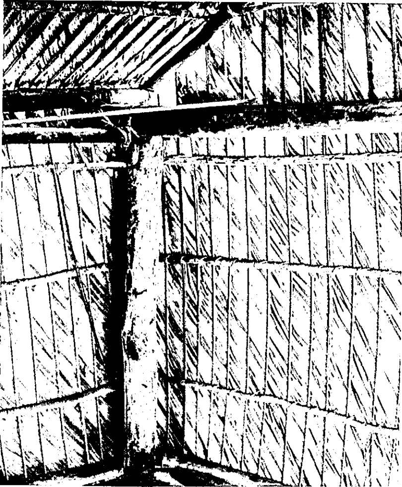
Detail of weather screen on the windward side of a Warao house.
